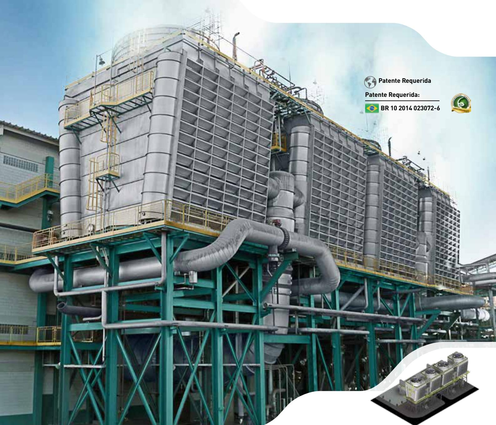
A large industrial evaporative condenser is shown from a low-angle perspective. It features a complex network of vertical heat exchanger cells with horizontal fins, supported by a green steel frame. Large, curved grey pipes connect the units. A yellow metal staircase and walkways are attached to the left side. In the bottom right corner, there is a smaller, 3D-style diagram of the same condenser unit.
